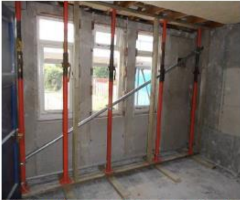
P7 – Ground floor propping (prior to erection of security screening)
