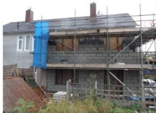
P12 – External Walls
